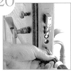
Install the armor front with the small phillips head screws supplied.
