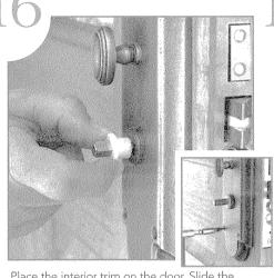
Place the interior trim on the door. Slide the aligning bushing onto the spindle so it fits into the knob hole. Drill pilot holes and fasten interior trim with supplied fasteners. Remove bushing and discard.
