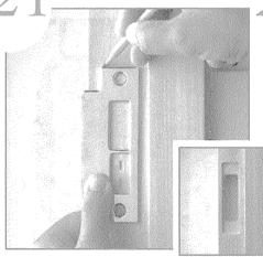
Mark the Jamb for the proper strike location. Coat extended latch bolt with graphite, powdered chalk or lipstick. Retract the bolt, close the door and actuate the knob or lever several times to mark the jamb. Add approximately 1/32" clearance from that mark.
