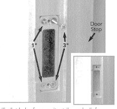
Drill pilot holes for security strike and relief holes for finished strike. Install dust box and security strike with 1" and 3" screws on the stop side of the plate. Note: Security Strikes are supplied only with locks which utilize cylinders.
