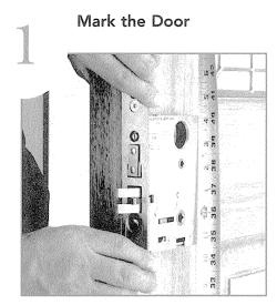
Mark the door at 37-1/2"- 40" above finished floor, or if retrofit, at appropriate location to coordinate with existing strike preparations. This will be center line of the lock and will put the knob/lever at 36" - 39" above the floor.
