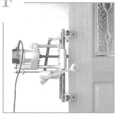
Mortise the pocket in the door 1/8" deeper than the lock being installed. Refer to the **Installation Template Guide Chart (blue sheet)** for exact size of mortise pocket.
