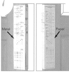
For 1-3/4" doors, fold the **yellow lock template** and attach to door using <u>Installation Template</u> <u>Guide</u>. Mark door at appropriate locations for lock and trim. **MARK APPROPRIATE BACKSET.**
