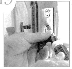
Tighten the cylinder set screw by turning clockwise. **Do not over tighten**. **Do not use** a **power screw driver**.
