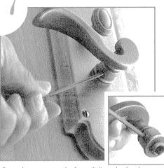
Start the set screw before sliding the knob or lever onto the spindle. Slide knob or lever onto the spindle and tighten securely. For knob to knob and lever to lever sets - install both sides - go to step 19.
